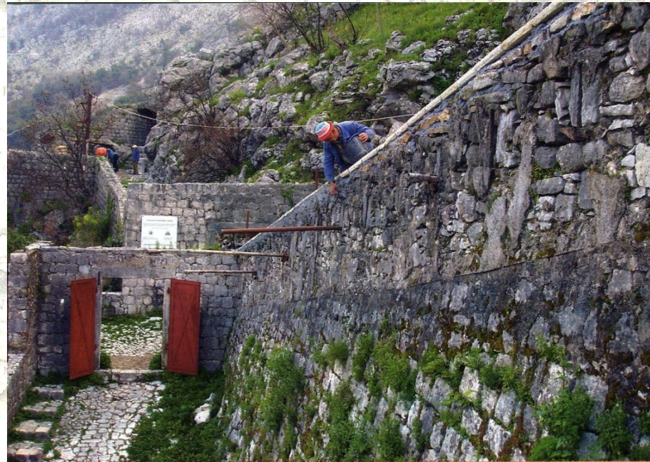
Reconstruction of cobblestones, steps, and ramparts of Kotor Fortress, Montenegro. U.S. Consulate in Podgorica, Serbia and Montenegro
